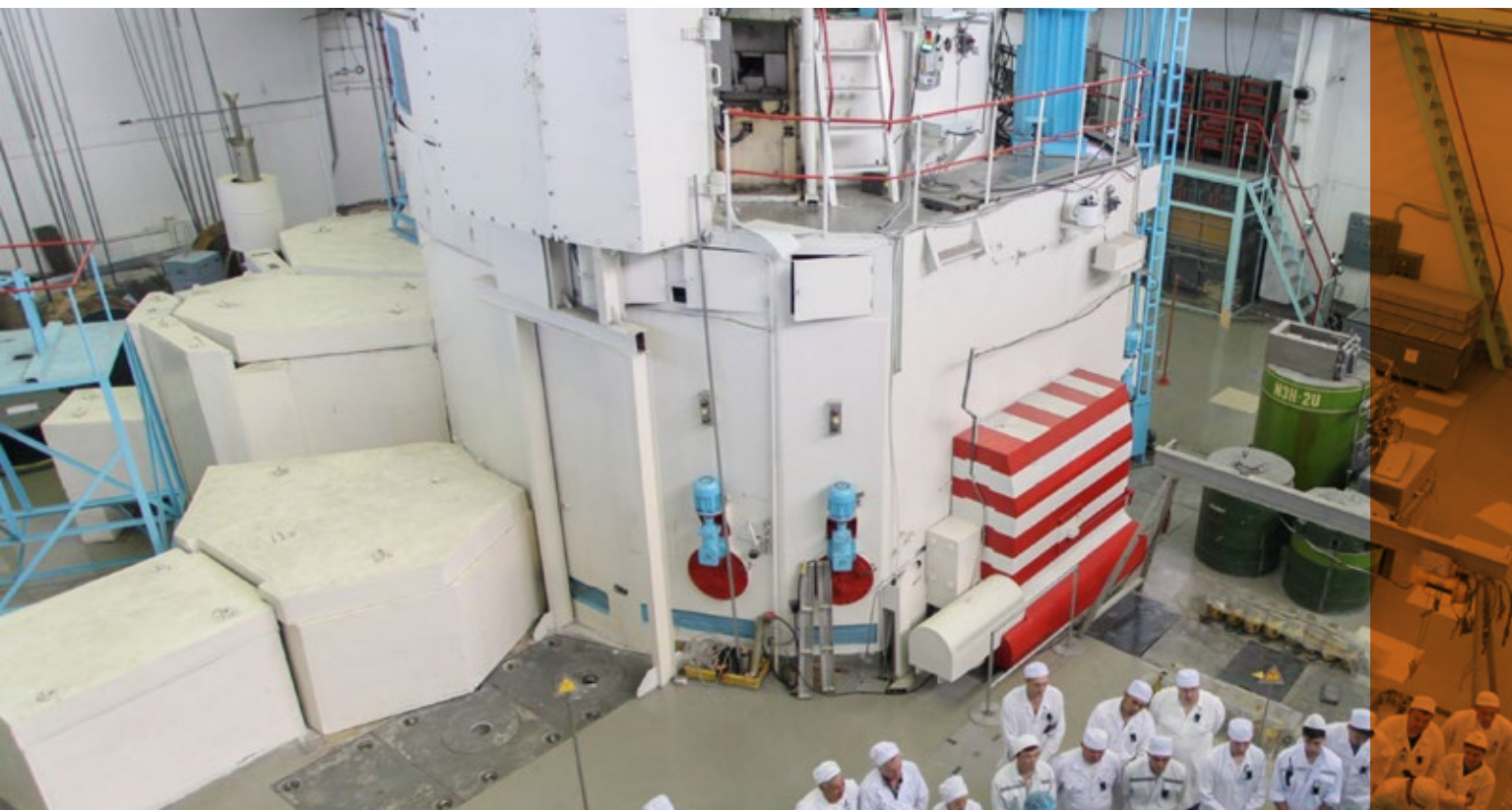
Argonne scientists worked with the Kazakh Institute of Nuclear Physics to convert their scientific reactor to run on less dangerous low-enriched uranium.
