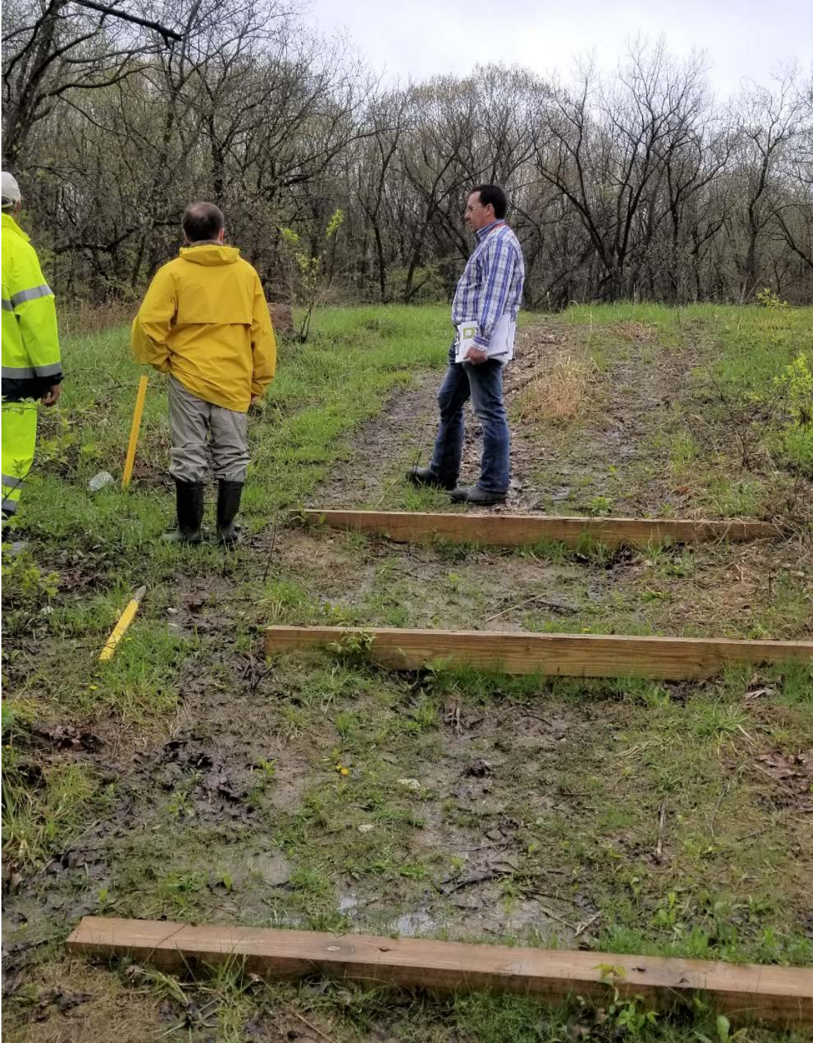
Figure 1.1 View of timber steps installed along northeast path at Plot M
