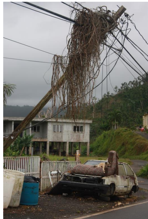
Figure 3: Downed Power Lines in Puerto Rico after Hurricane Maria (photograph by Jane Palmer)
