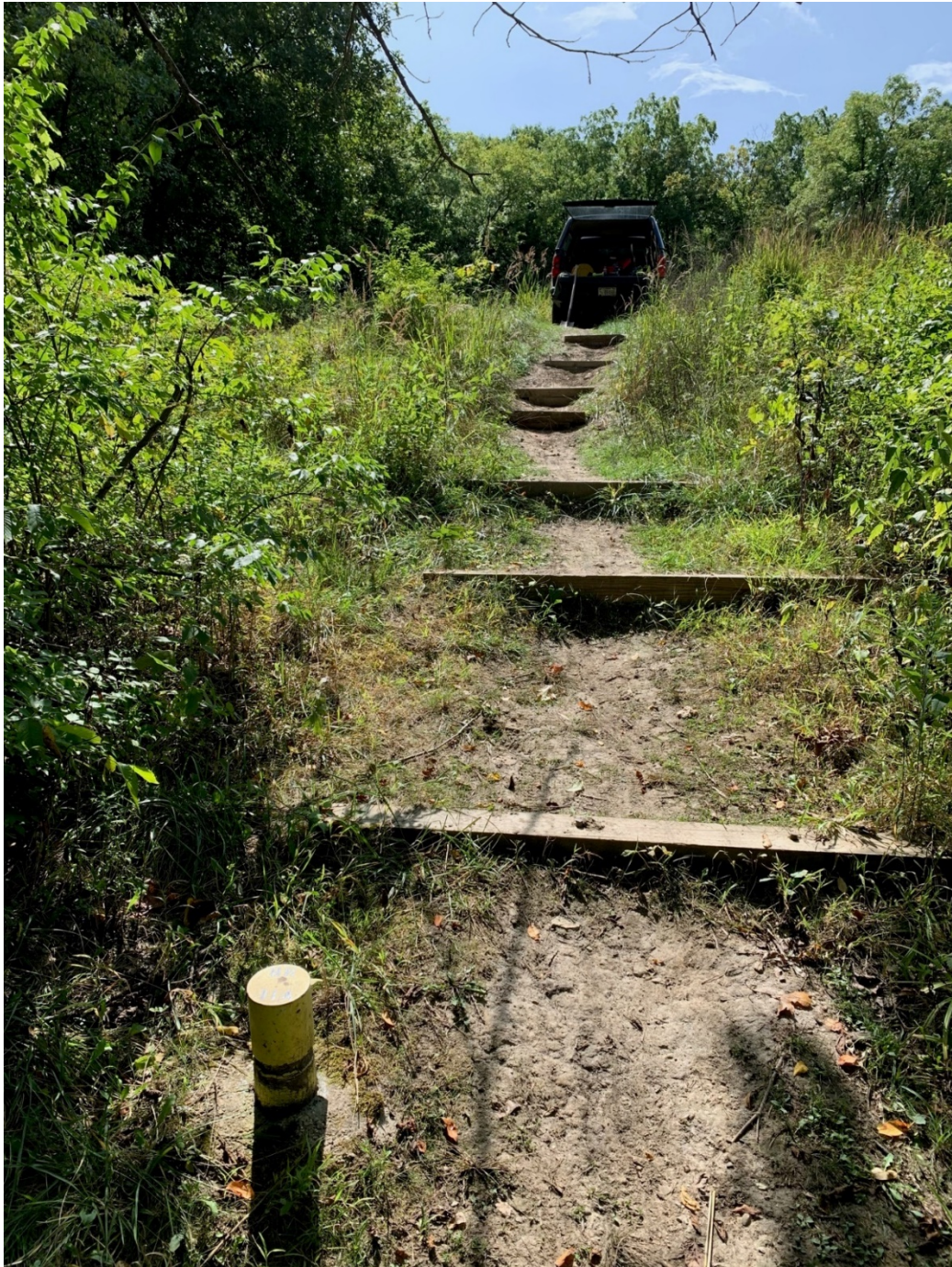
Figure 1.3 View of Timber steps at Plot M and BH#11.
