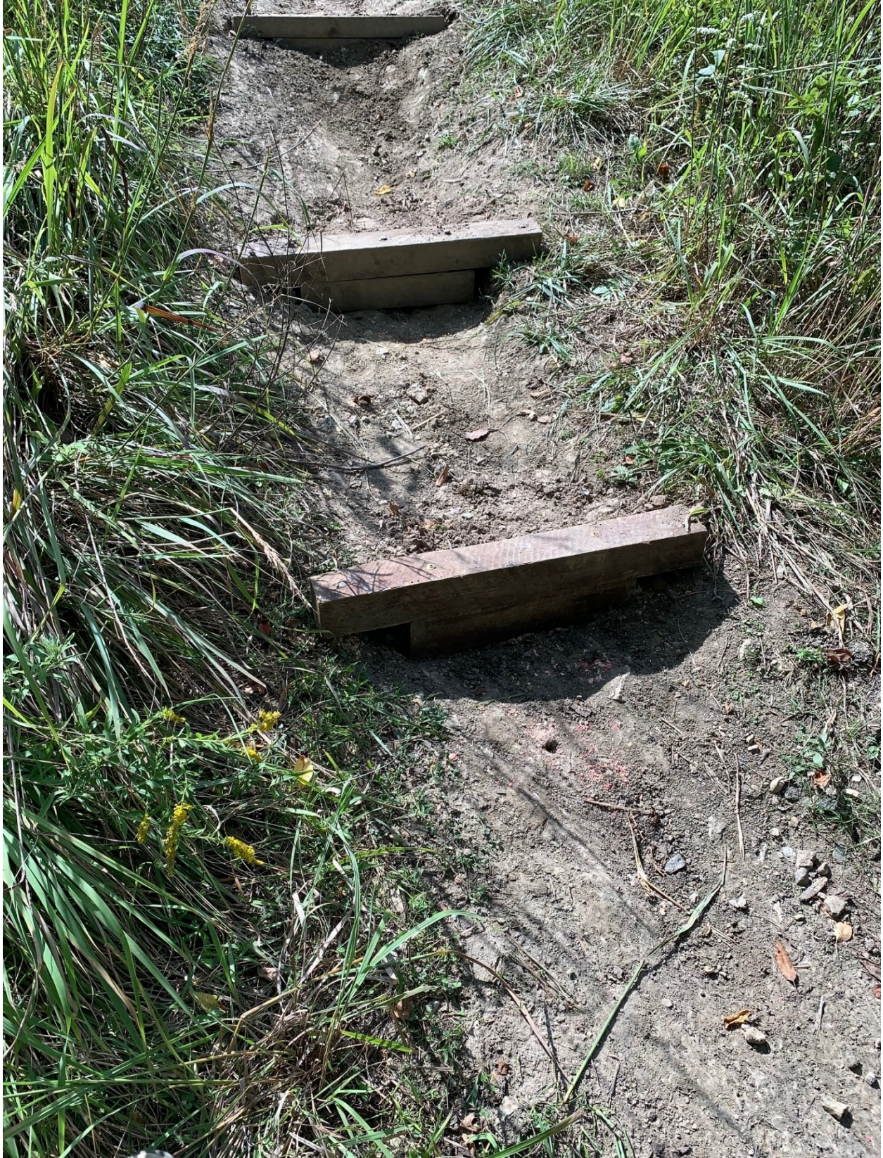
Figure 1.2 View of timber steps installed along northeast path at Plot M.
