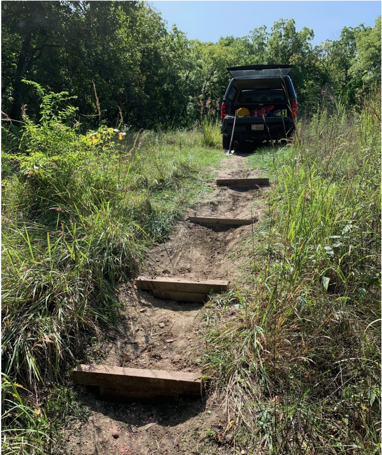
Figure 1.1 View of timber steps installed along northeast path at Plot M.
