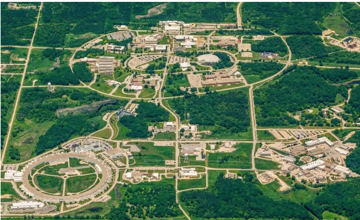
Figure 1. Aerial view of the Argonne site today. Photo credit: Argonne National Laboratory.
